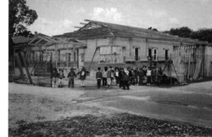
The Pre Primaries visit the New Administration Block site.
